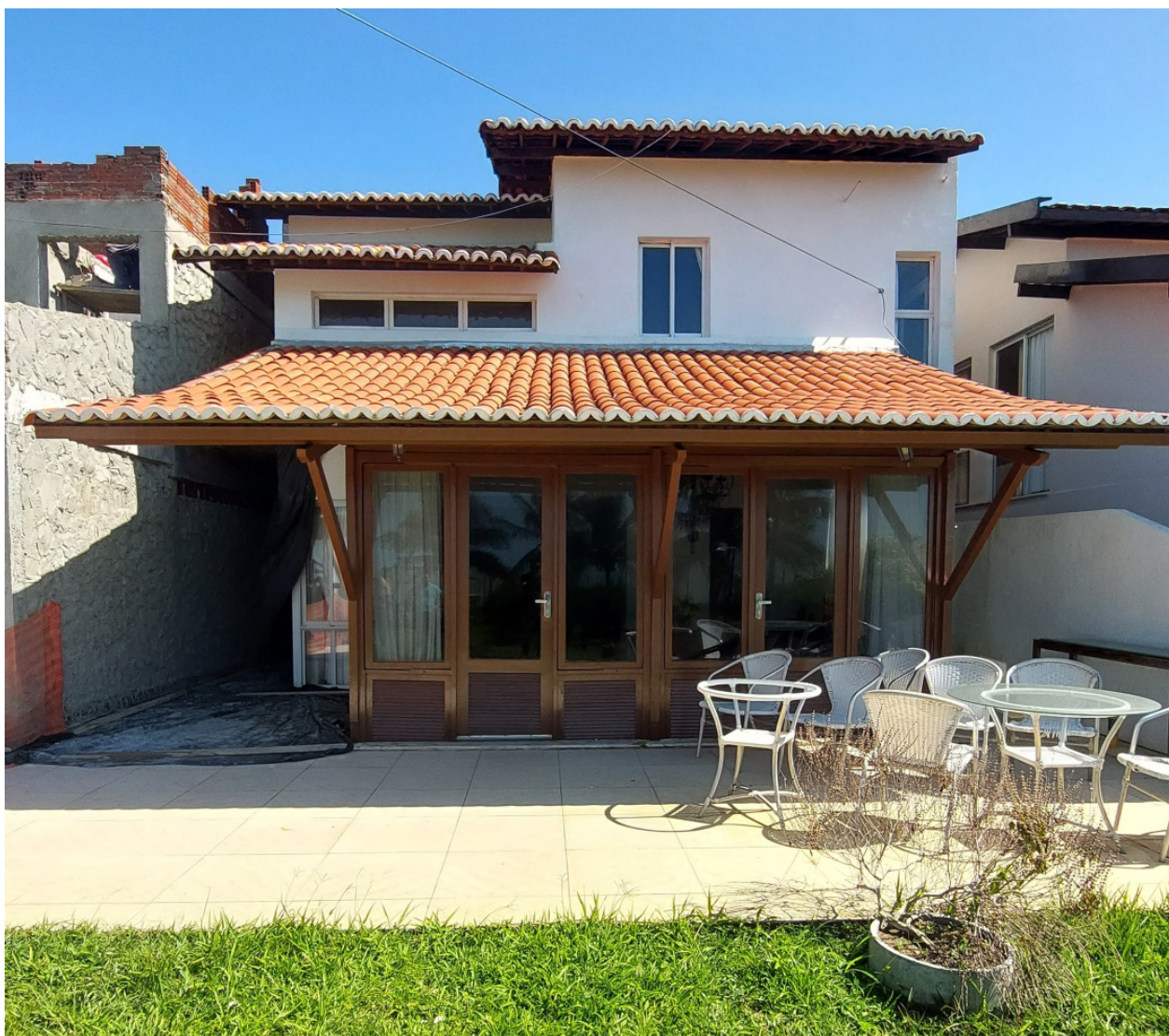
Vistoria in loco
