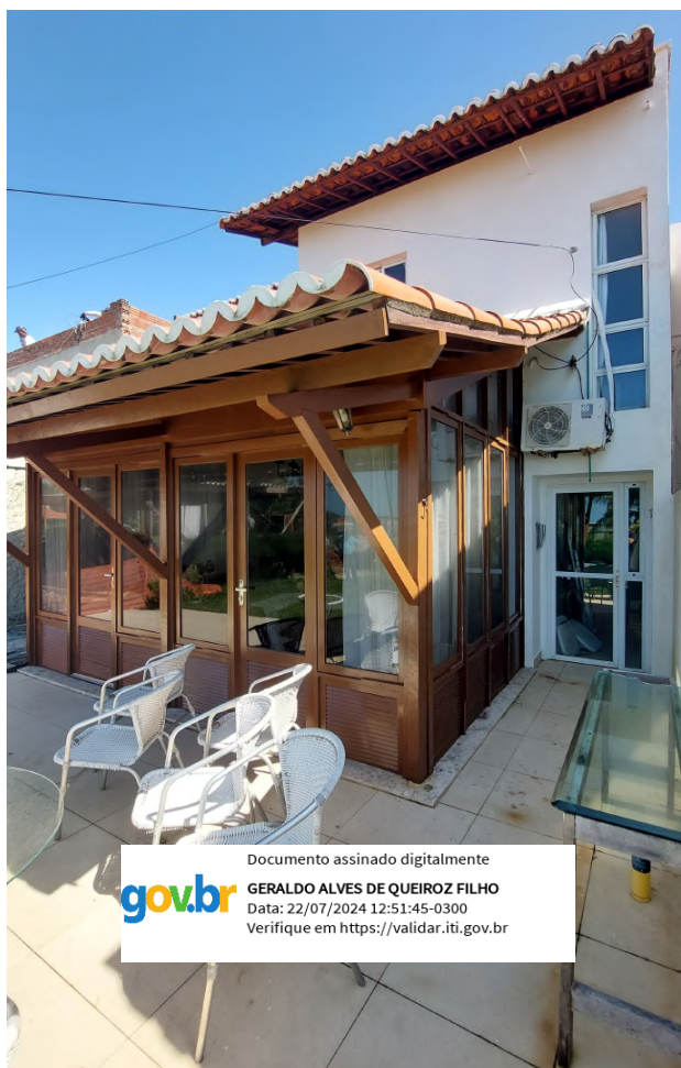
Vistoria in loco
