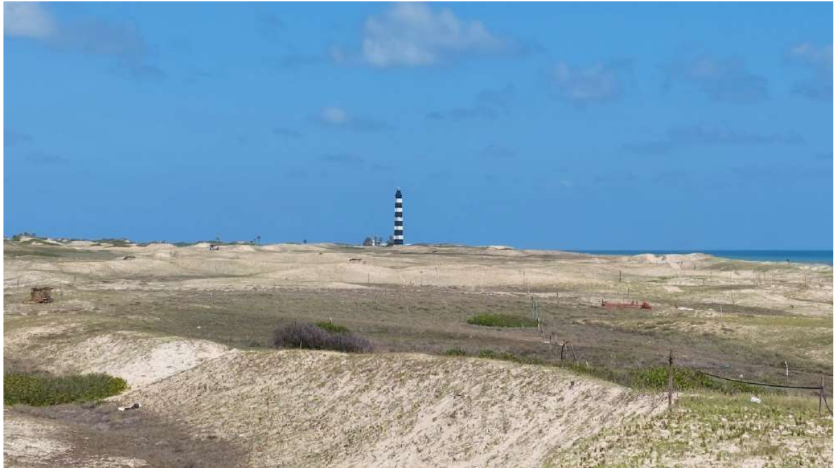
Vistoria in loco
